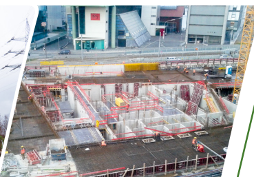
Construction site in Düsseldorf's harbour district
